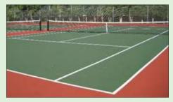
The four tennis courts are now nearly completed with the resurfacing which takes place over a 5 - week period from the week of 12 October to 16 November 2015 during which period they have to be closed. The 5 - week closure period is to allow the new porous tarmac surface to properly "cure" before its surface is painted.
