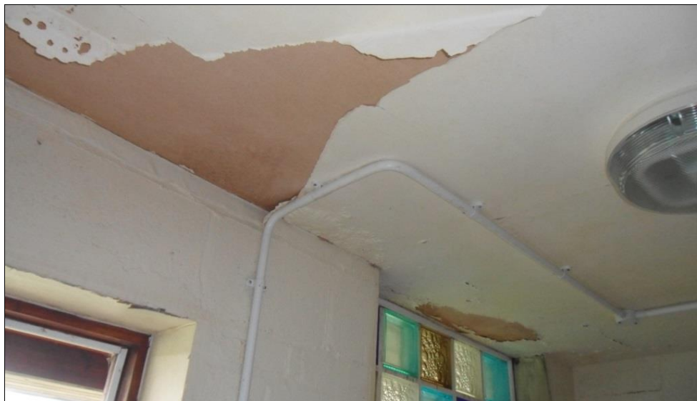
Fig 4 Internal view within existing pavilion
