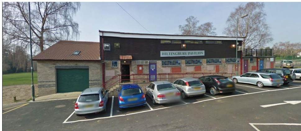
Fig 3 Existing pavilion – © Google Street View
